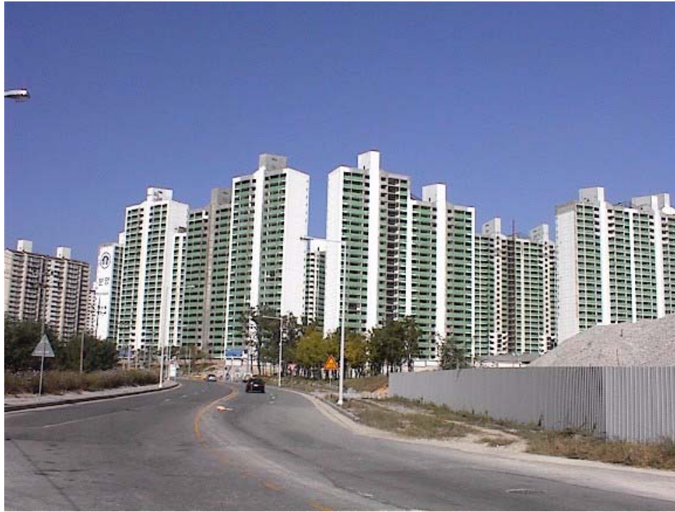
Exurban Residential Development Under Construction (North of City)
