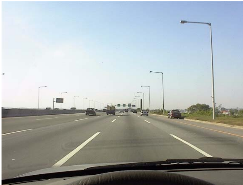
Motorway on North Bank of the Han River
